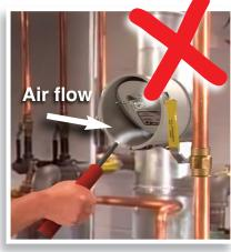
Tankless coil boilers waste fuel through draft regulators.
