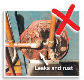
Tankless coil boilers typically fail at the coil flange or cast iron sections. *Ascent has no coil flange or cast iron sections.*
